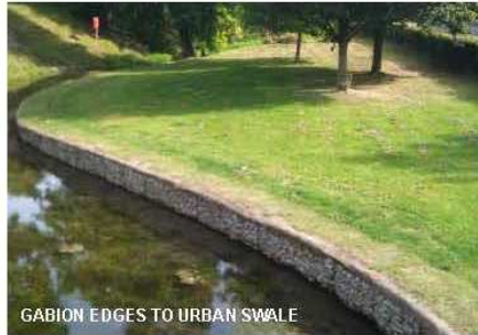
GABION EDGES TO URBAN SWALE
