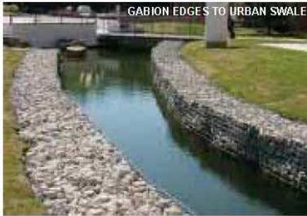
GABION EDGES TO URBAN SWALE
